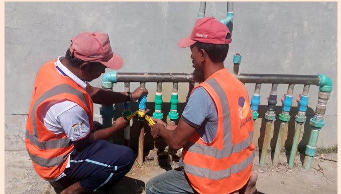
Ongoing WASH Maintenance work
